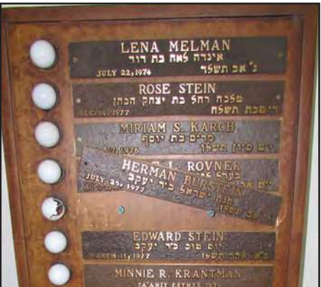
Close-up of one of the side panels prior to restoration showing a loose plate, broken bulb, light damaged wood and chipped paint.
