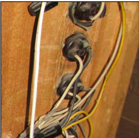
Outdated and potentially dangerous wiring prior to restoration
